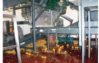
Existing installation with conveyors under juicing machine.
